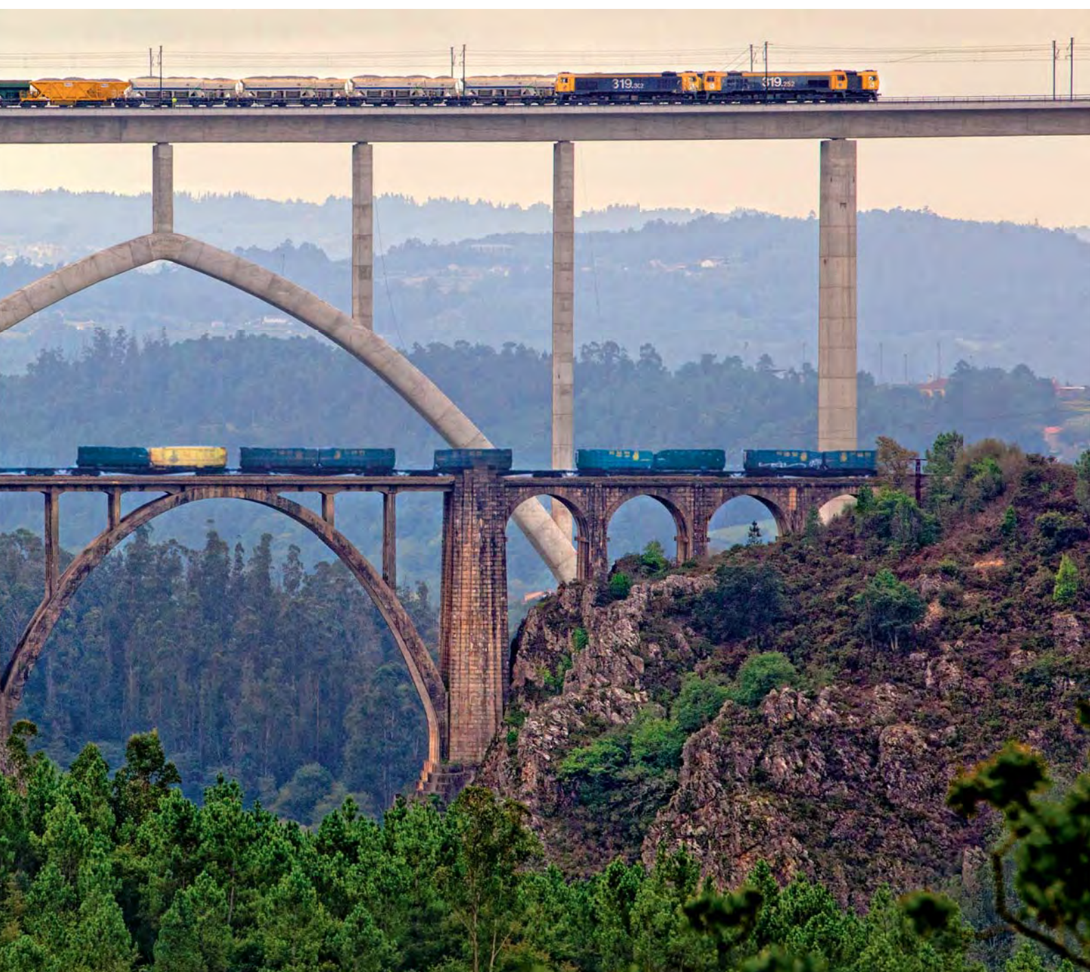
Cover photo: Viaduct over Ulla river, Madrid-Galicia high-speed railway line (Spain).
